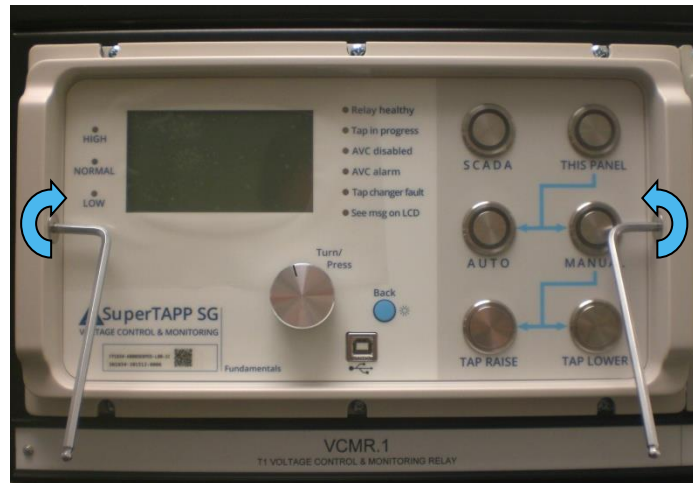
Figure 1-5 Installing the relay
