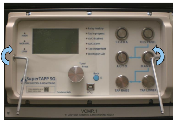
Figure 1-34 Replacing the relay
